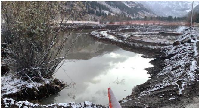
Tailings area NTN has been fully excavated and the drainage channel flowing through it has been restored.
